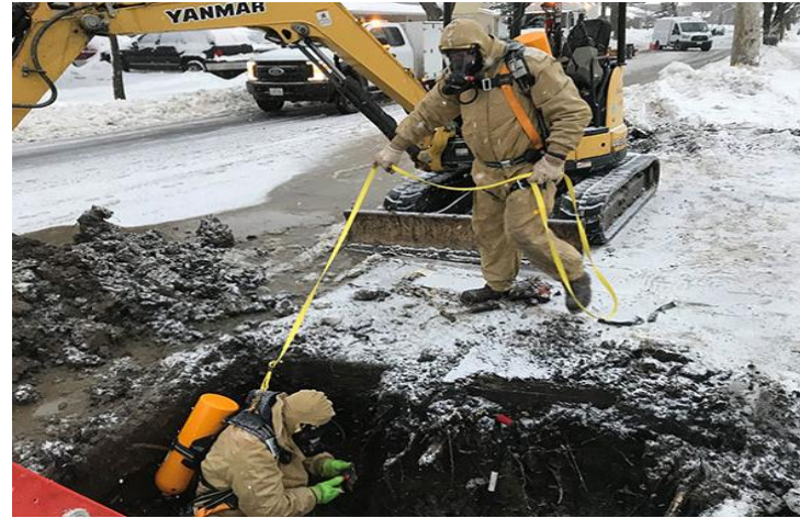
Repairing damage caused by water main break
